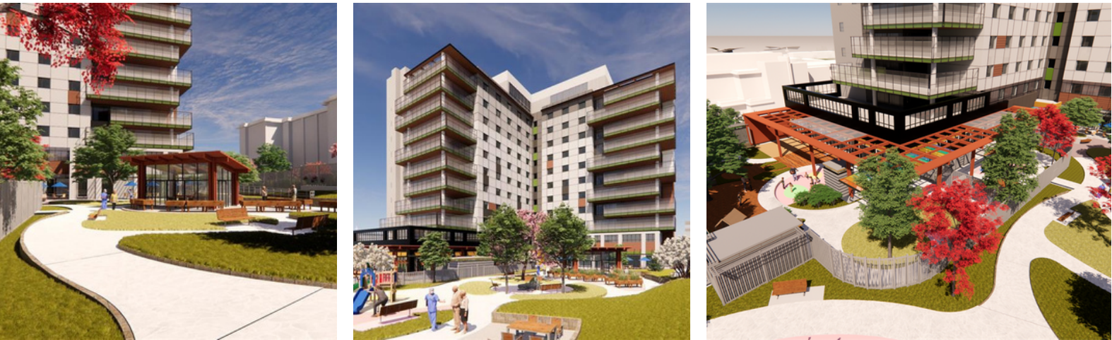
Construction is underway for the new St. Vincent’s: Heather long-term care home, set to welcome 240 residents in late 2028. Located at 33rd and Heather, the 13-storey facility builds on the success of Providence Living at The Views in Comox, bringing its innovative care village model to Vancouver.
