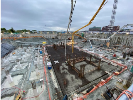
Concrete pumps and crews pouring concrete at the new hospital (June 2022).
